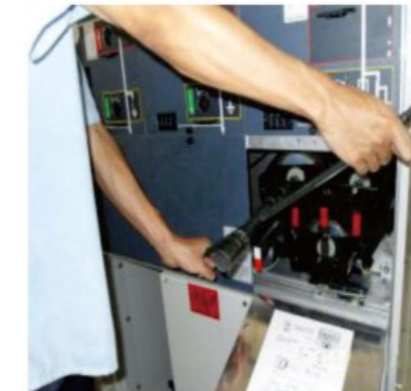
⑤Rotate counterclockwise with the operating handle to open the fuse unit.
