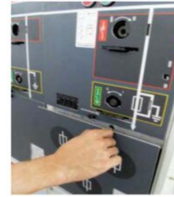
③Loosen the panel in fuse room. ④Incline the panel in fuse room, in order to operate fuse unit.
