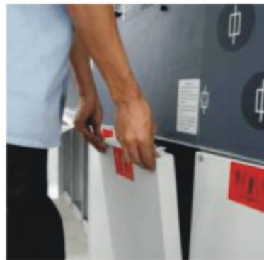
Loosen the screw of cover plate of cable chamber, take out the cover plate and remove
