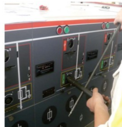
②Rotate the operating handle clockwise to close the earthing switch
