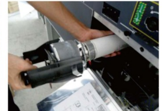
⑥Pull the handle of fuse unit. The fuse is fixed on the box cover of the fuse tightly.
